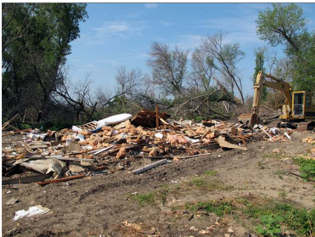
Fig. 3. The final demolition in progress. Photo credit: Dale Wrubleski.
