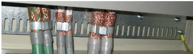
Figure 6.2: Screen termination at earth strip.
