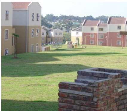
Figure 2: Three-storey walk-ups in Amalinda with the communal area in the centre
