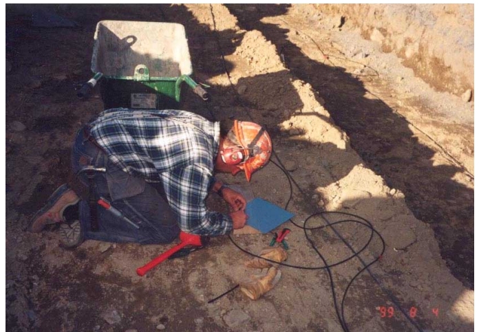
Figure 4. Installation of resistivity electrodes.
