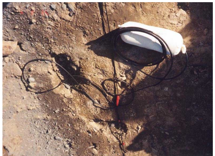
Figure 5. Installation of SP electrodes.
