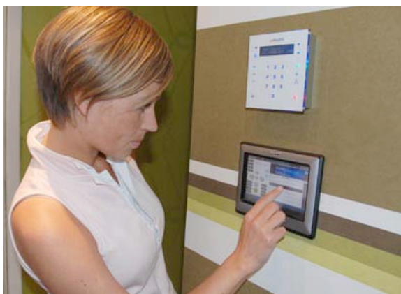
Fig.15: Air-conditioning and light control panel in the Smart Home [53]
