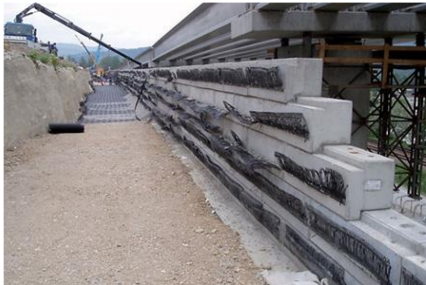
Fig. 3: Installation of reinforcing geogrids on the reverse side of facing blocks.
