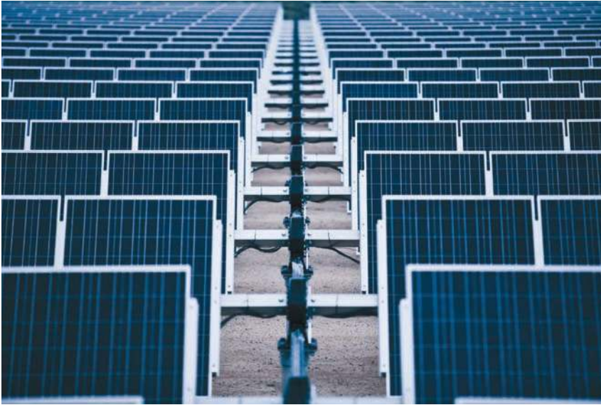
Solar energy in New Mexico contributes to mitigate climate change.
