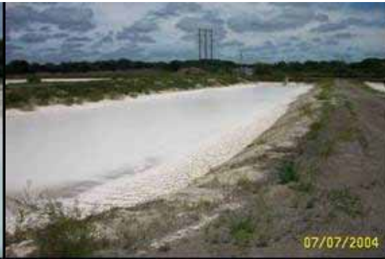
Figure 3: Dewatering Lagoon after 3 months settling
