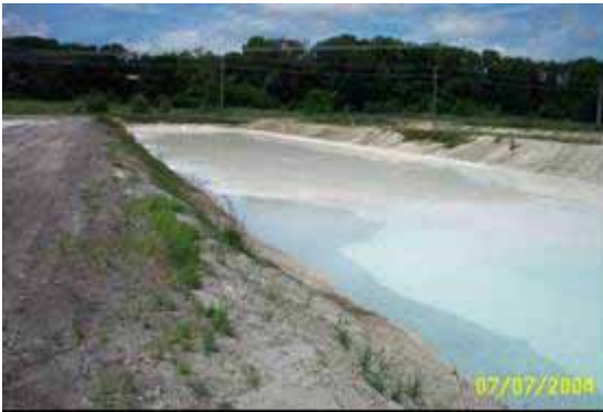
Figure 2: Dewatering lagoon while filling (looking towards the end from which the sludge enters)
