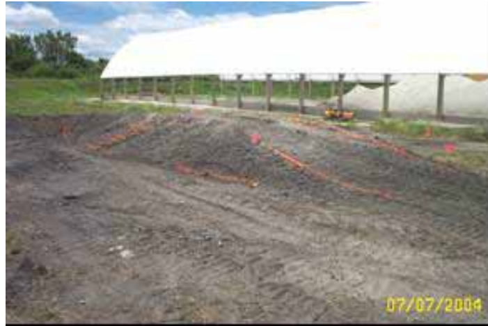
Figure 39: Test embankment with topsoil cover after 7 days
