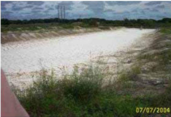
Figure 4: Dewatering lagoon after 10 months settling
