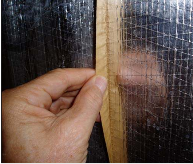
Figure 5–8. Noncontacting Overlap Between Insulation Sheets
