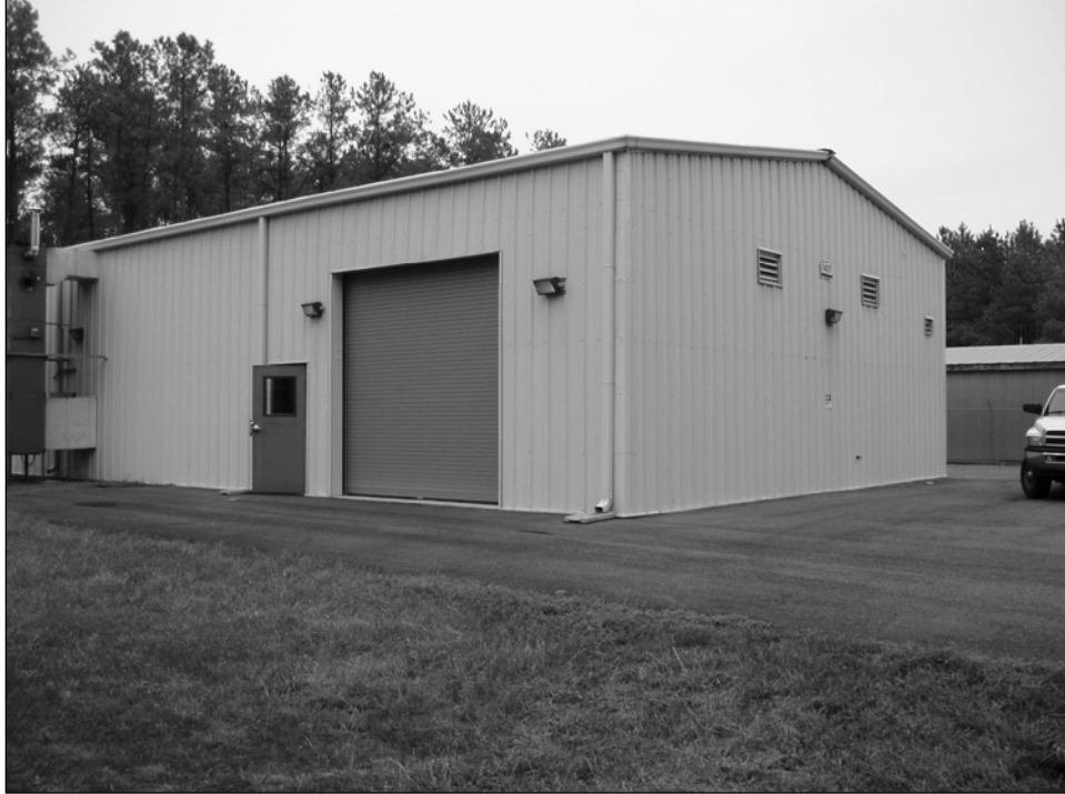
Figure 4–2. South End of Building 1427 Showing the West Overhead Roll-up Door
