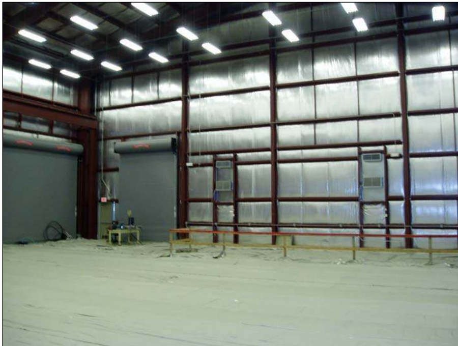
Figure 5-4. ERG Building Interior with Covered Floor
