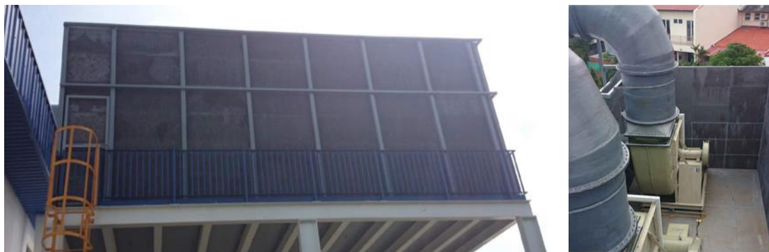
Figure 7. Industrial application in a factory extension as a noise barrier
