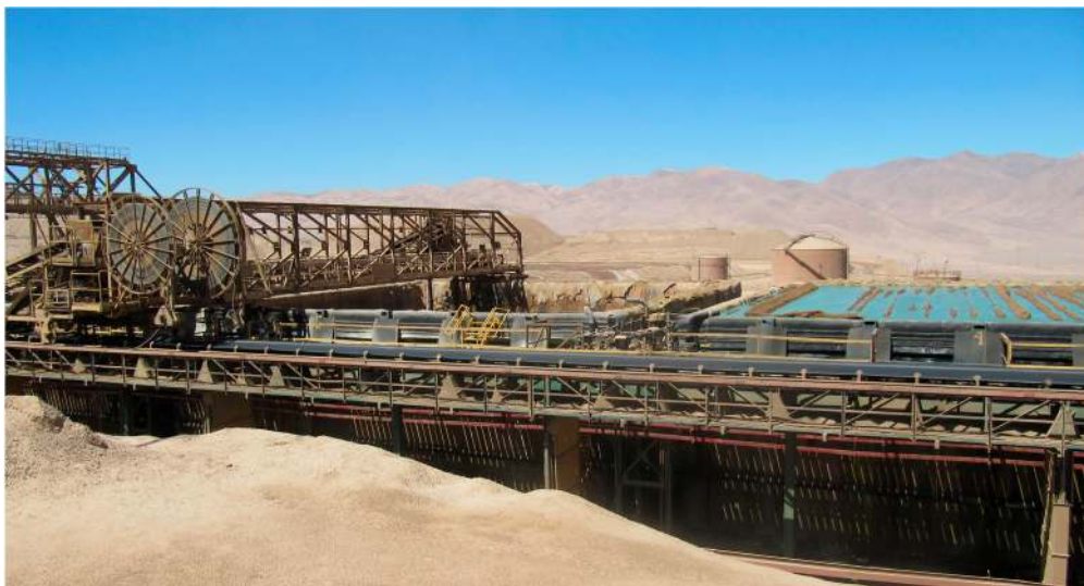
Figure 4. Vat leaching of oxidised copper ore at Mantos Blancos, Chile. Photograph by D.W. Shiers, reproduced with permission.
