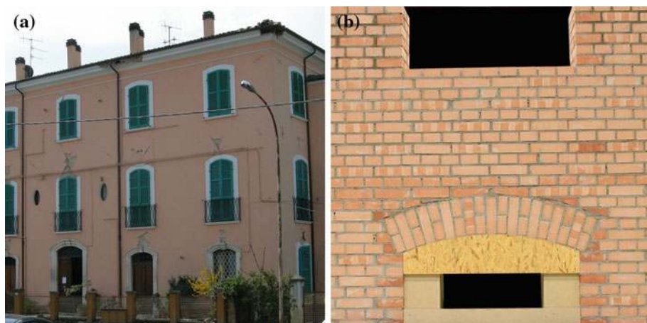
Fig. 1 Old URM building during the L'Aquila earthquake on April 6th, 2009, showing spandrel failure a and detail of a spandrel test unit ( b , Beyer and Dazio 2012a )
