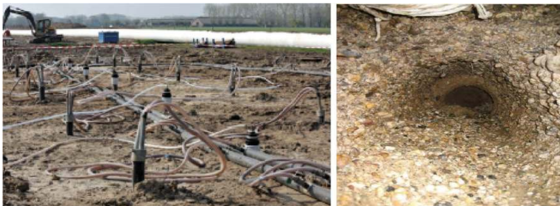
Fig. 5 First field application of MICP. (After: [7], with permission from ASCE)
