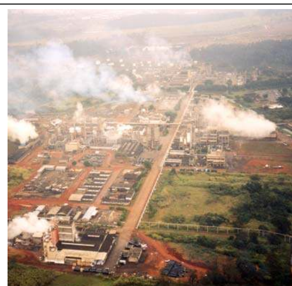
The smelter complex in Kitwe
