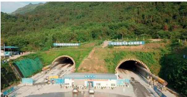
FIGURE 2: The construction site of Case 7 during the lockdown (source: http://www.zgjt.com/zhitong/2020-05/29/content_243523.htm ).
