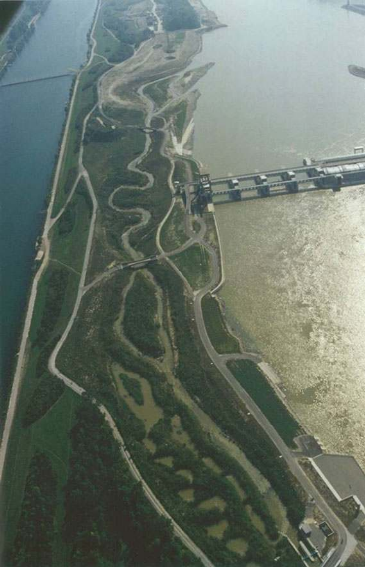
Fig. 24.7 Bypass channel system for fish migration at the power station “Freudenau” (Section 4) (courtesy of Verbund AG)
