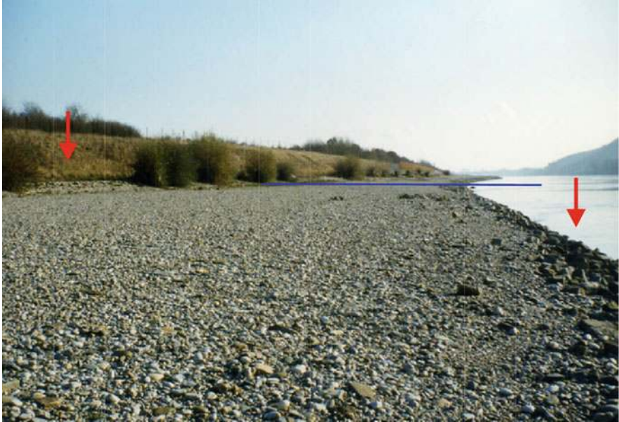
Fig. 24.5 Extended underwater gravel bank inshore structure under construction; red arrows indicate “double riprap”; blue line indicates the water level nowadays after construction (Section 2)
