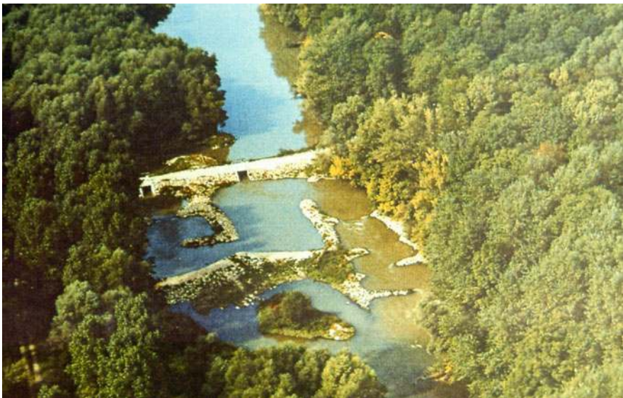
Fig. 24.4 Lateral connection of Korneuburger Au with the main channel of the Danube via a fish bypass system (courtesy of Verbund AG)
