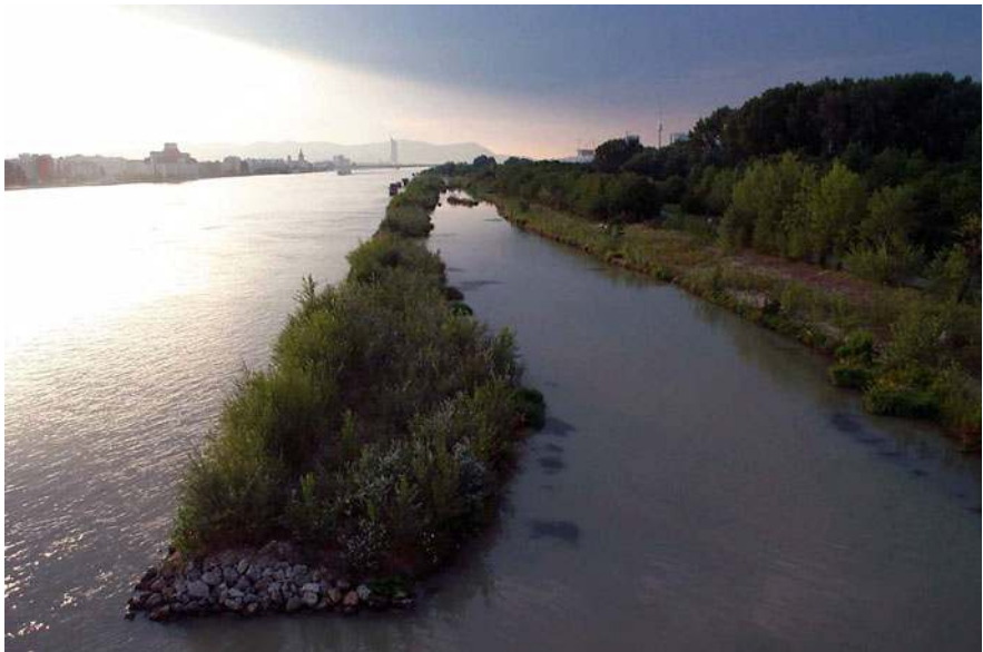
Fig. 24.6 Constructed riparian channel and bay system in the central impoundment (Section 3)
