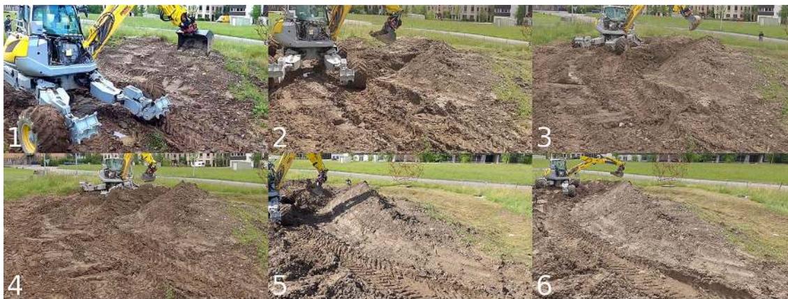
Fig. 15 A time-lapse with six images over the entire fabrication process shows the progress of the s-curved embankment
