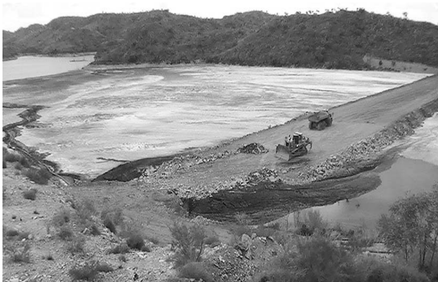
Figure 17 Groyne No. 9 near completion to full height
