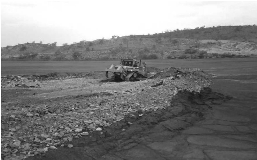
Figure 16 Mud wave ahead of D10
