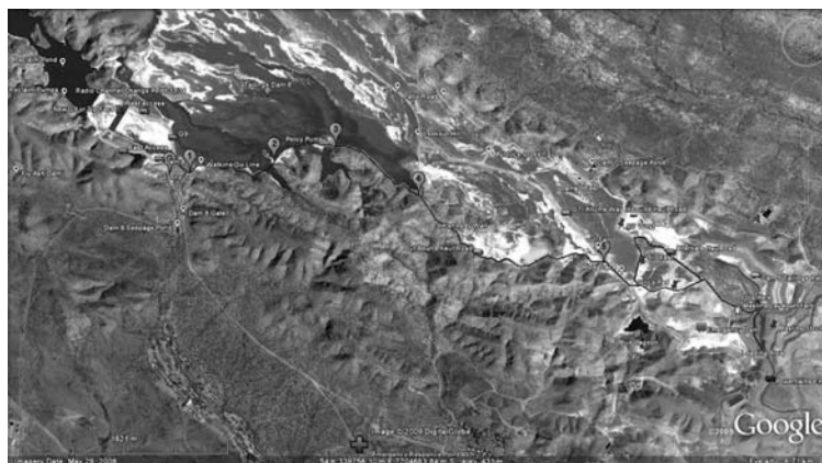
Figure 1 Tailings storage general layout (north to left border)
