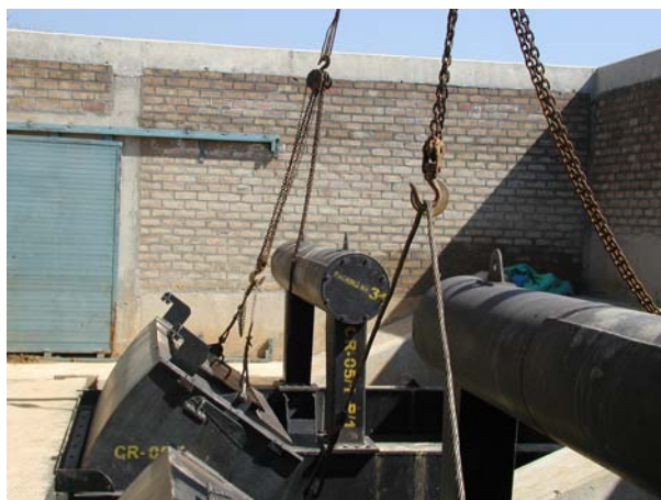
Figure 9.7. Use of chain pulley to control flow in the Maira Branch Canal
