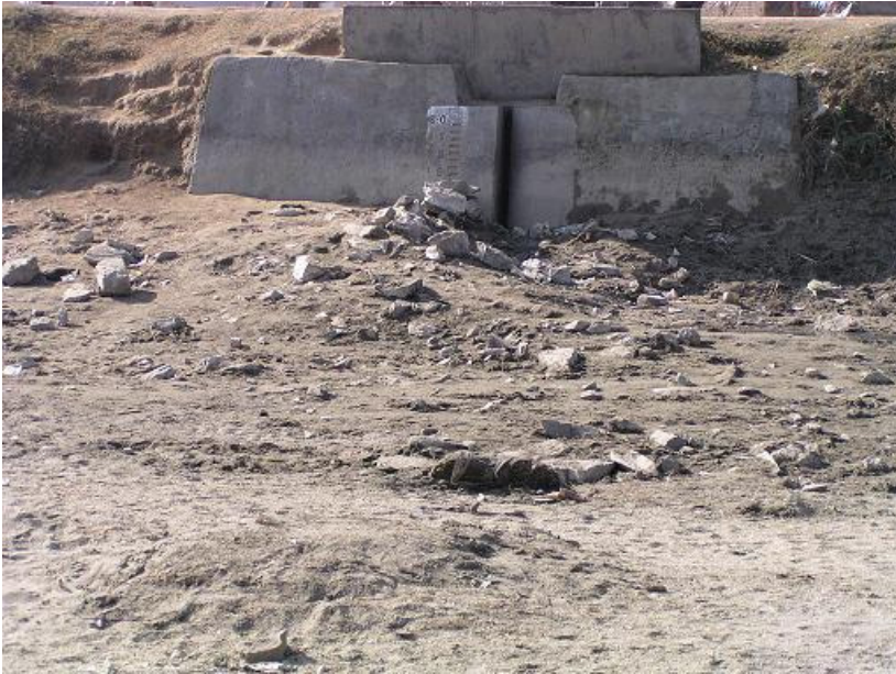
Figure 9.4. Sedimentation in front of an outlet
