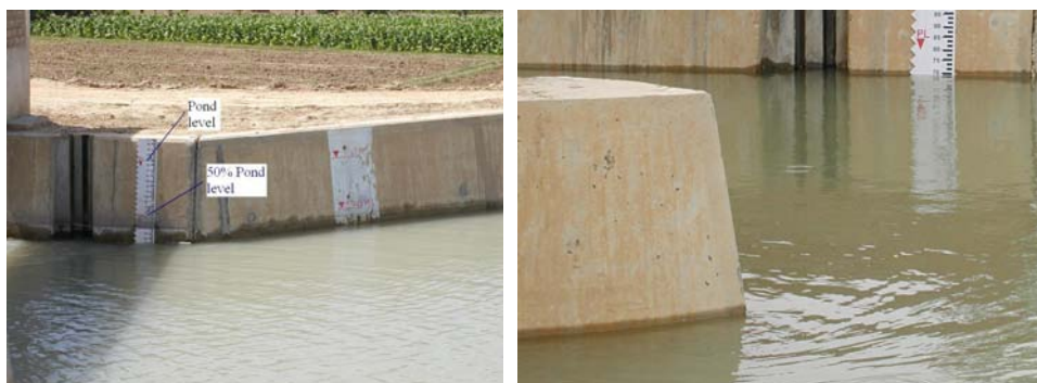
A. Water level at high discharge
