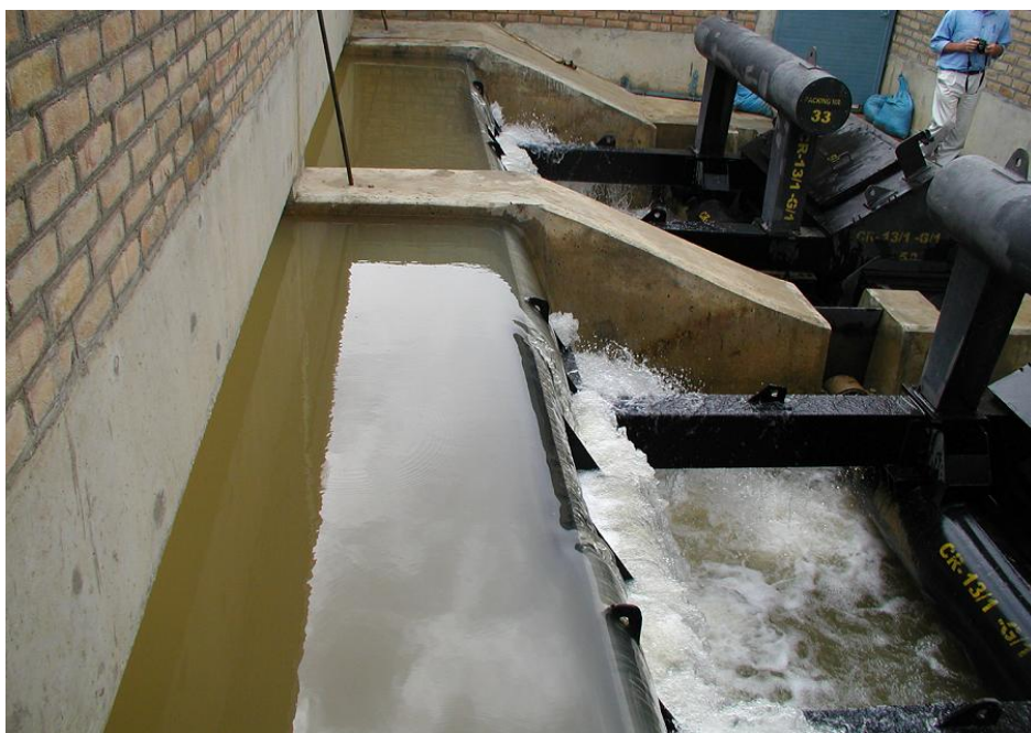
Figure 3.12. Overtopping of the AVIS gates in Maira Branch Canal, Pakistan
