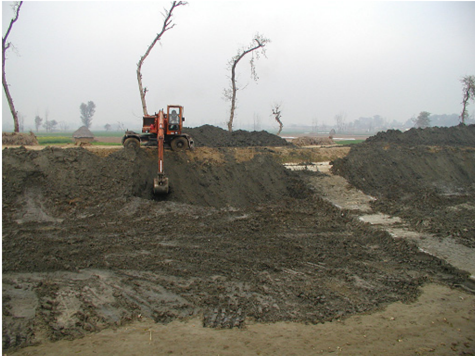
Figure 9.3. Desilting of Lower Machai Branch Canal in January 2007
