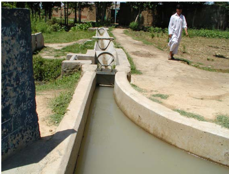
Figure 9.14.A. Closure of tertiary outlet by a refusal gate by farmers
