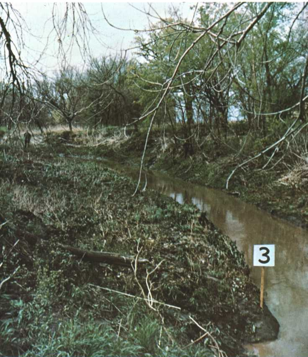
No. 825 downstream from below section 2, Salt Creek at Roca, Nebr.
