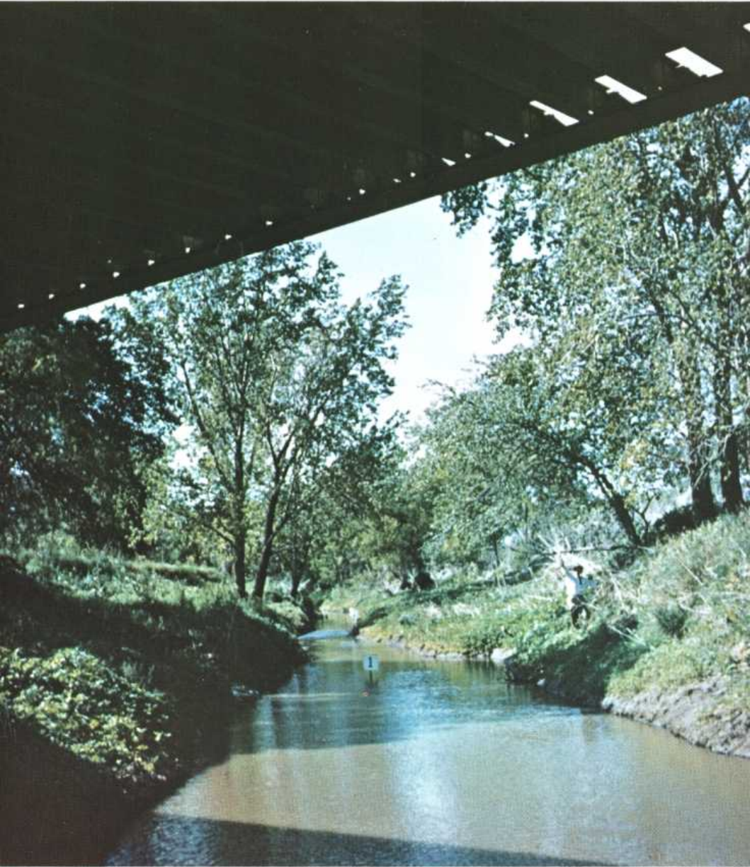
No. 824 downstream from above section 1, Salt Creek at Roca, Nebr.
