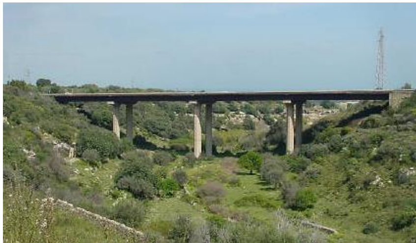
Figure 13. West side elevation of the Cusumano bridge
