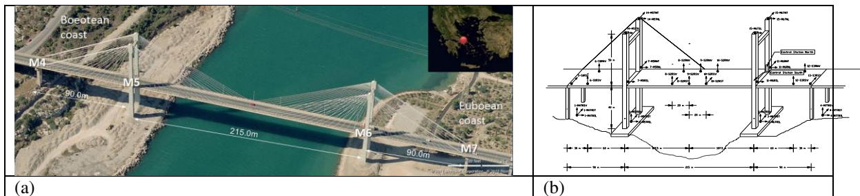
Figure 26. (a) The Cable-stayed section of the Evripos Channel bridge (b) instrumentation layout
