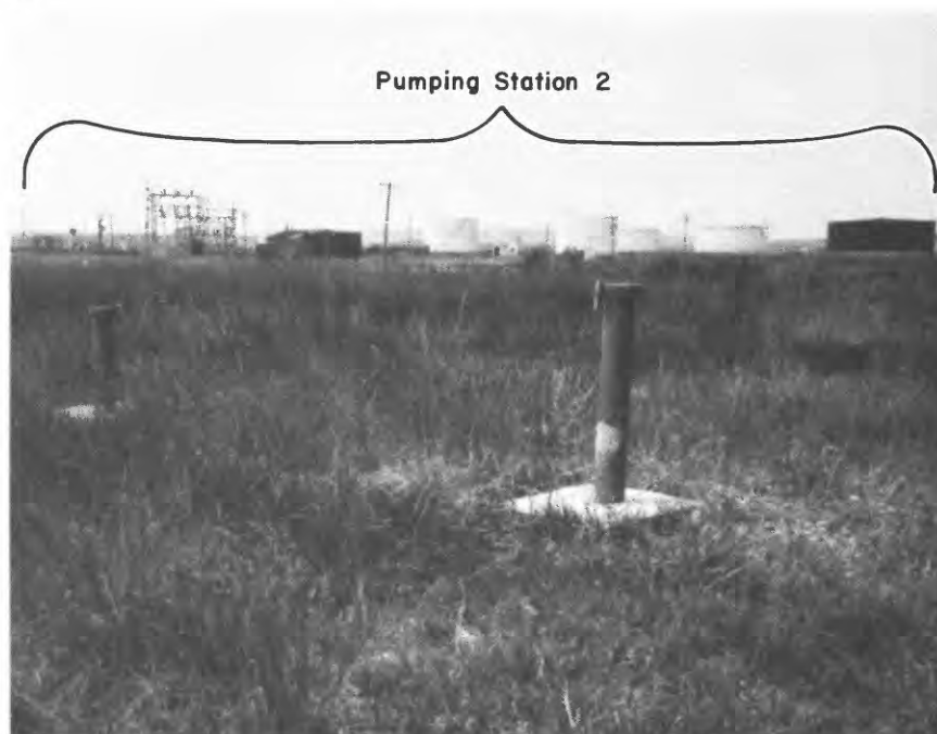
Figure 3. Various surface structures associated with oil production in the East Poplar oil field study area, northeastern Montana. (A) View east (from NE 1/4 NW 1/4 SE 1/4 SE 1/4, sec. 19, T. 29 N., R. 51 E.) of a brine-injection well (Murphy 5-D; pl. 3), and an evaporation pit (behind pump house). (B) View northwest (from NE 1/4 NW 1/4 NW 1/4 NW 1/4, sec. 32, T. 29 N., R. 51 E.) of monitoring wells (FPB92-1 and FPB93-2; Thamke and others, 1996, table 1) near storage tank facilities (Pumping Station 2).
