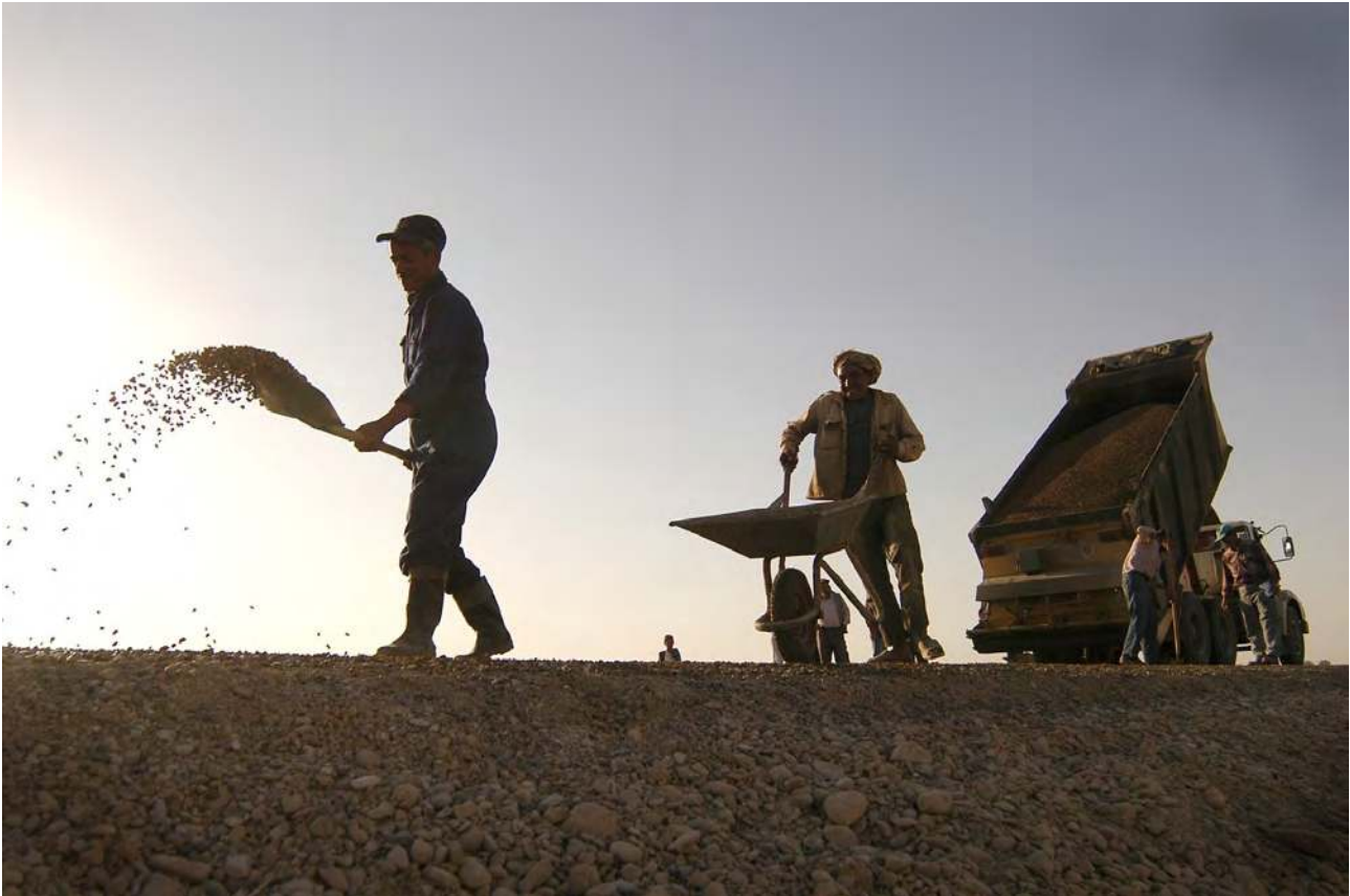
Workers on a road construction site
