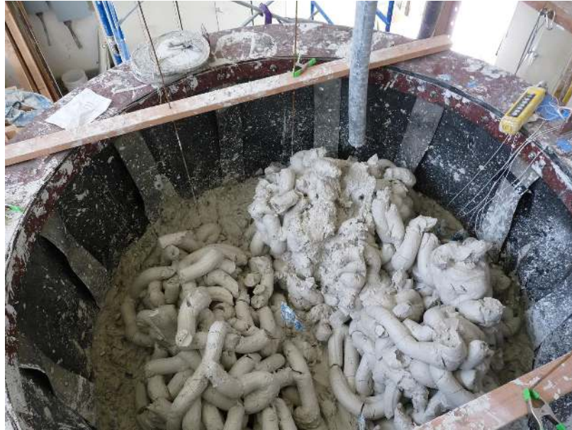
Figure 4.9 - Material immediately after discharge from mixer, ready to be hand packed
