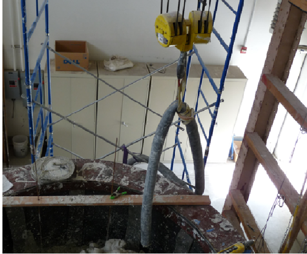
Figure A.6 - Discharge hose held and controlled using the overhead crane
