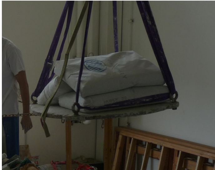
Figure A.5 - Platform hung from crane for transporting material
