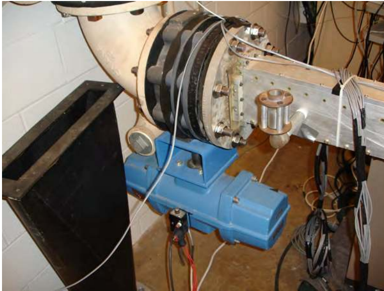
Figure F.18: Vacuum chamber solenoid valve and controller
