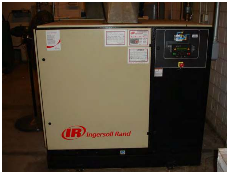
Figure F.3: Ingersoll Rand rotary screw compressor
