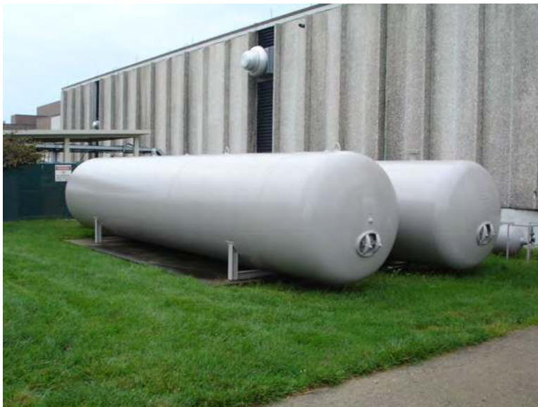
Figure F.5: High pressure and vacuum chambers
