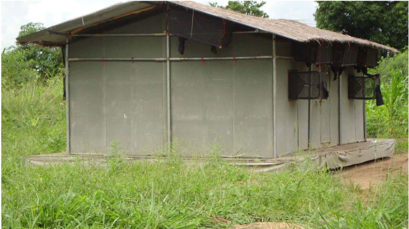
Figure 2. A wooden experimental hut. The experimental huts were designed to represent local housing in southern Tanzania. An experimental hut had a corrugated roof and covered with grass thatch on the top, to simulate the temperature of local houses with thatched roofing. The outer walls were constructed from wooden planks or canvas. The inner walls were made of removable panels coated with mud. They had one door and two functional windows with open eaves (open spaces between the roof and the walls). doi:10.1371/journal.pntd.0000773.g002
