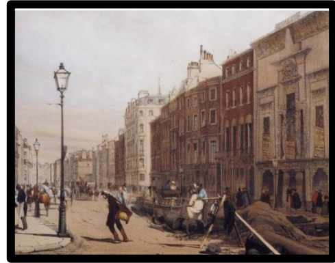
Figure 15: Webb, R. (2001) Installing the sewer system in between the Quadrant
