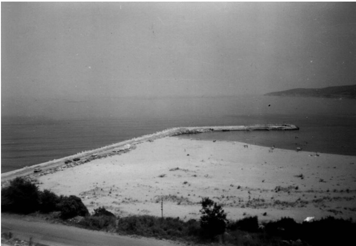
Figure 5: Sedimentation in the fishing harbour of Alepu
