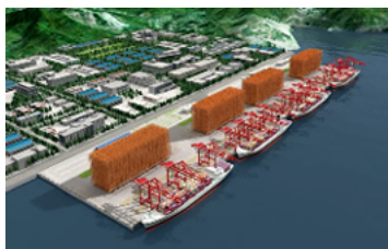
(a) Ultra-high container warehouse system (Source: Ez-Indus)
