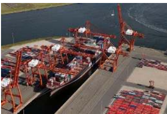
(a) Indented berth with QCs at both sides (Source: Young, 2012)
