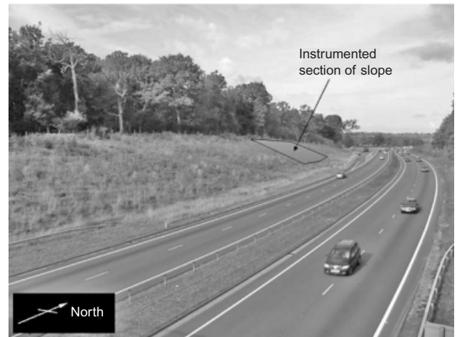
Fig. 2. Photograph of site
