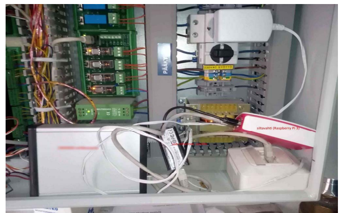
Fig. 1. Bridge device capturing traffic at a building
