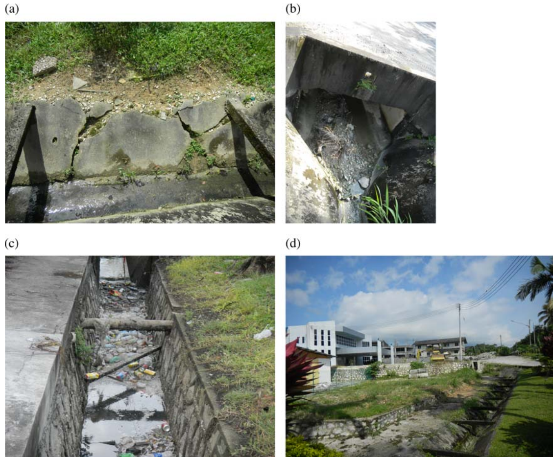
Figure 9. Factors affecting sediment deposition in urban concrete drains: (a) deteriorating drain condition such as broken drain at a site at Serian Residential releasing surrounding soil into drain; (b) design of the drain where changes in cross-section especially under culvert at a site at Serian Commercial will cause sediment deposition; (c) blockage due to garbage downstream such as a site at Mak Mandin Industrial and (d) too near to source of aggregate for example construction/renovation site such as a site at Serian Commercial where aggregate will go into nearby drains.
