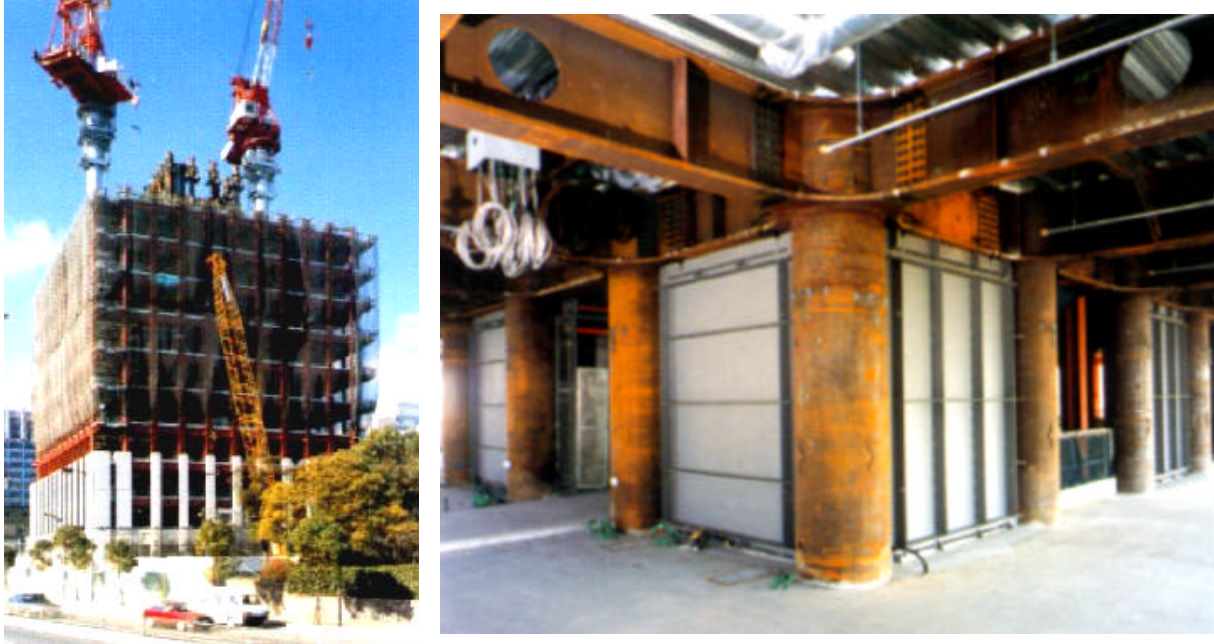
Figure 2.14. A view of building with Low Yield Point (LYP) steel plate shear walls and a close-up of the walls
