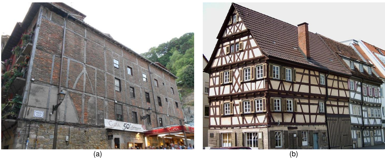
Fig. 1 Examples of timber frame buildings: (a) historic buildings in calle 31 de Agosto, San Sebastián, Spain; (b) typical timber frame buildings in Sindelfinge, Baden-Württemberg, Germany
