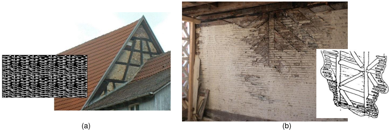
Fig. 3 Types of infill: (a) willow basketry in Germany (Bostenaru 2004); (b) taipa de fasquio in Guimarães and adoption of same infill for frontal wall (Mascarenhas 2004)
