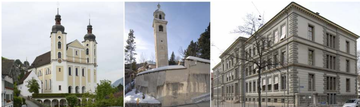
Figure 5. Three examples of cultural heritage buildings in Switzerland: Church St. Peter and Paul in Sarnen OW (Category A, left), Leaning Tower of St. Moritz GR (Category B, center), and Blaesi school building in Basel (Category C, right)
