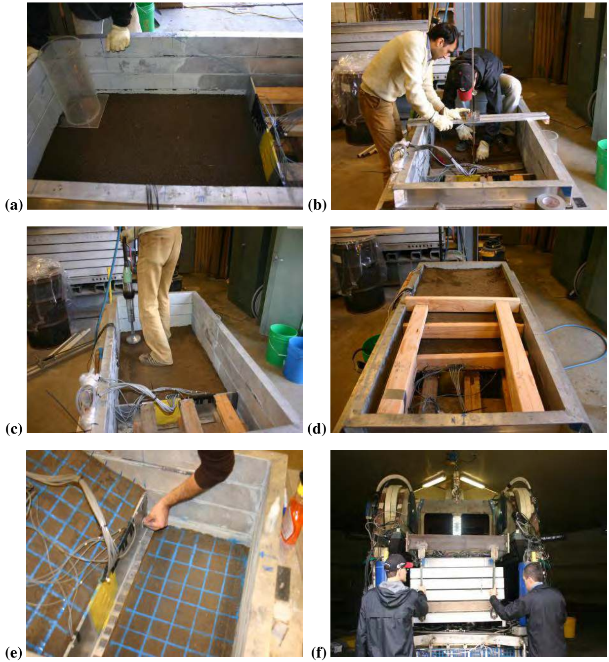
Figure 3.12 Construction of sloping backfill model GC02 a) placement of backfill, b) installation of accelerometers, c) pneumatic hammer compaction, d) wood struts used to prevent lateral displacements during compaction, e) finished slope, f) model in the arm.
