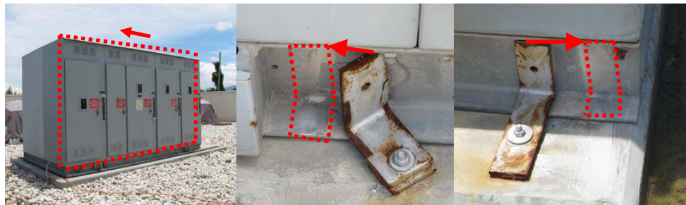
(b) Outdoor Electrical Cabinets – Sliding
