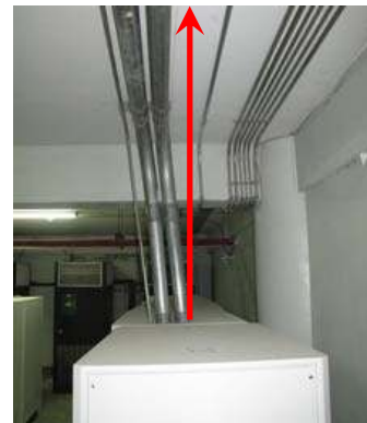
(b) Conduit at top of UPS at Digicel
