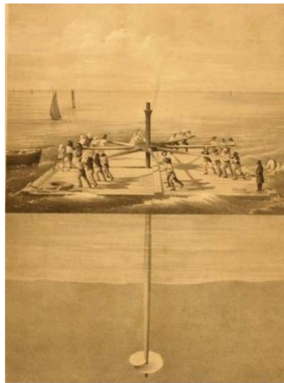
Figure 2-1: Labor installing Helical pile manually by applying torque – After Lutenegeger (2011)
