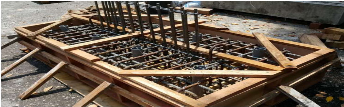
Fig.2. Preparation of foundation beam cage
