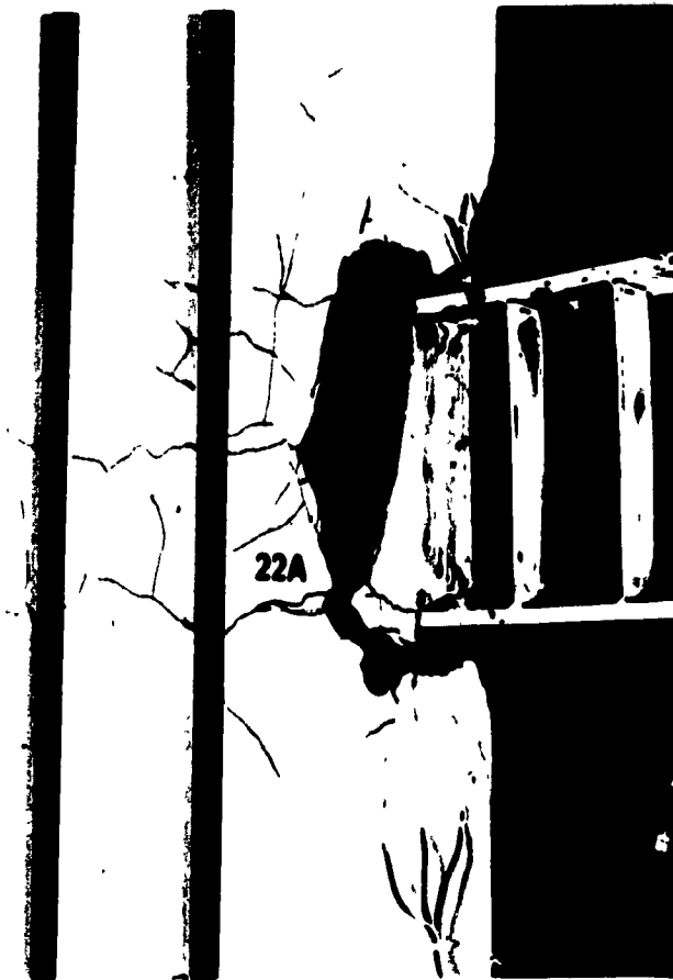
Figure 5.23 West embedment region of Specimen 2 at peak load 22A
