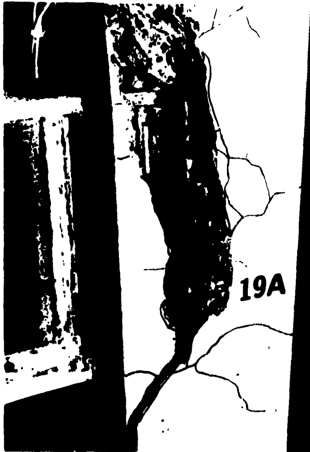
Figure 5.20 Vertical plane of cracking at east embedment region of Specimen 2 at peak load 19A
