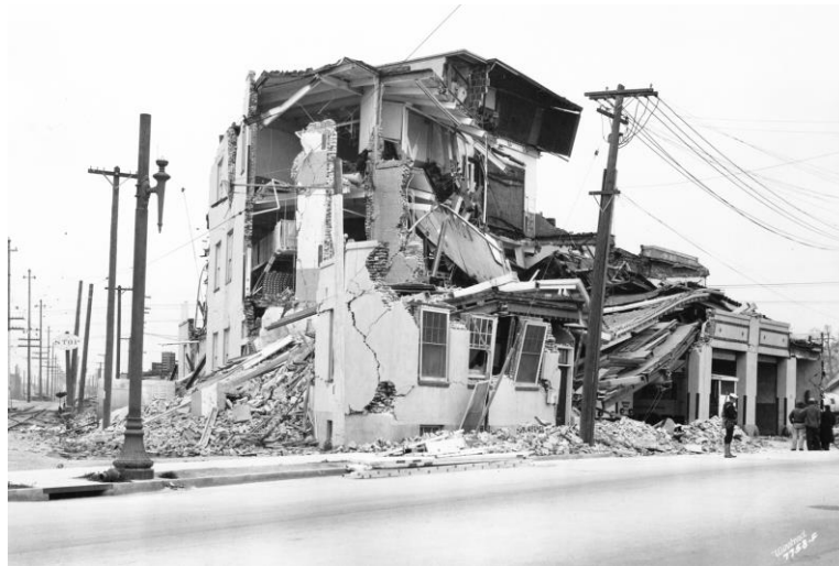
Figure 1-1: Complete Collapse of a Commercial URM building, Long beach, California 1933
