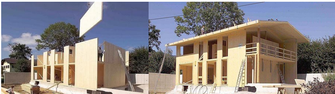
Figure 1-6: Cross Laminated Timber Building (KLH GmbH, 2010)
