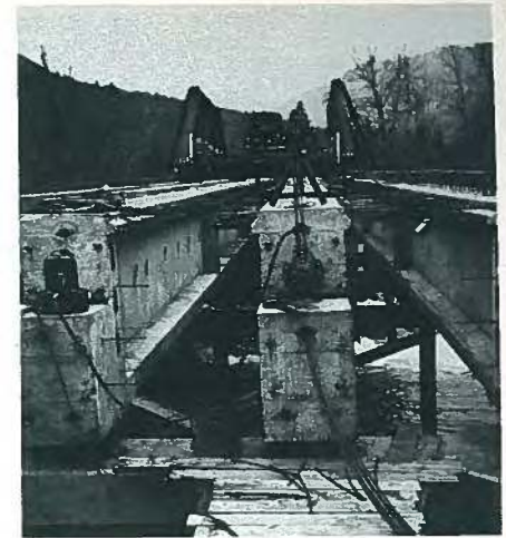
Fig. 79. Anderson post-tensioning system jack in position on Klickitat County bridge girder.
