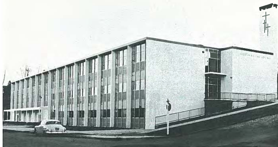
Fig. 67. Completed school, after only 6 months of construction.
