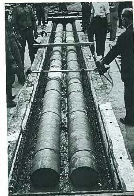
Fig. 20. Girder is about half cast, showing paper tubes used to form voids in the concrete.
