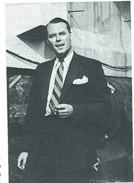
Fig. 2. Clement Atchit, resident engineer from Bleton-Aubert, Brussels. His know-how and friendly advice was a major factor in the successful production of the Walnut Lane test girder. In the background can be seen the prototype girder and steel ingots.
