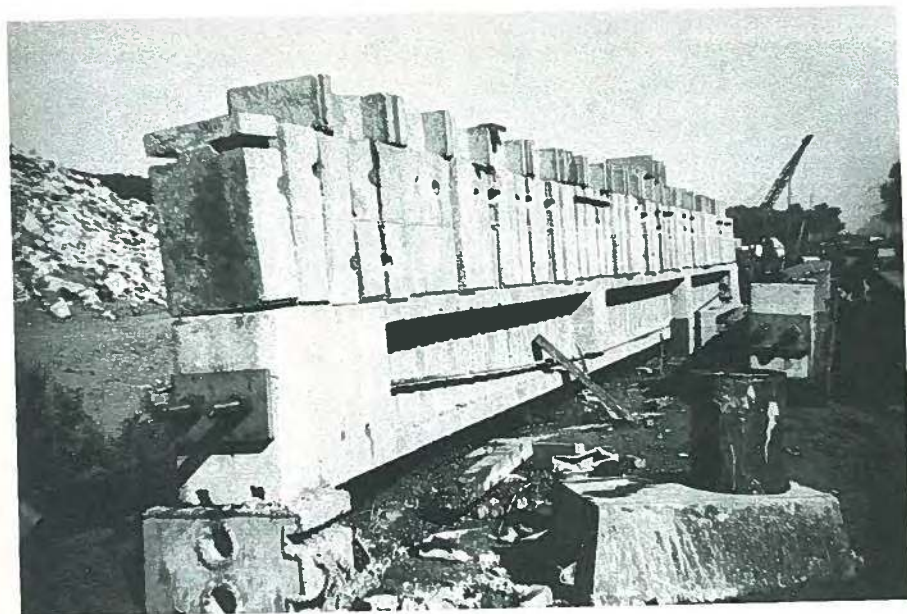
Fig. 15. Testing of Michigan block-beam with 1.5 live load.
