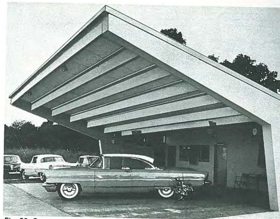
Fig. 20. Canopy using prestressed tee-joists and tectum roof deck. At one time in the mid-fifties this roofing system was quite popular in Florida but soon gave way to the double-tee.
