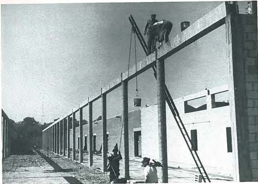
Fig. 12. Grouting continuity steel in 12 x 16-in. (305 x 406 mm) block beams of 40,000 sq ft (3720 m 2 ) warehouse for General Shoe Corporation.
