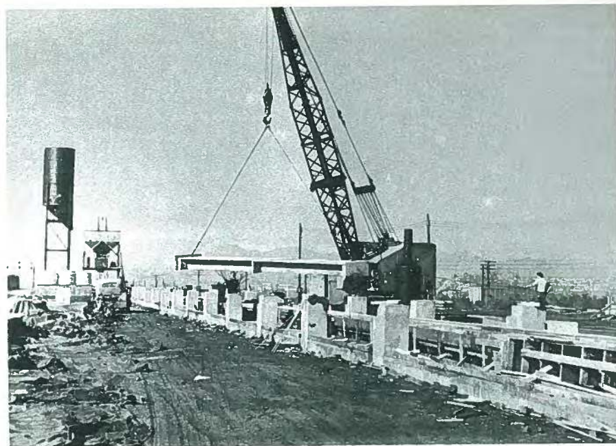
Fig. 11. A single-tee slab is lifted off the bed ready for transport to the Spitzer Electric Company.
