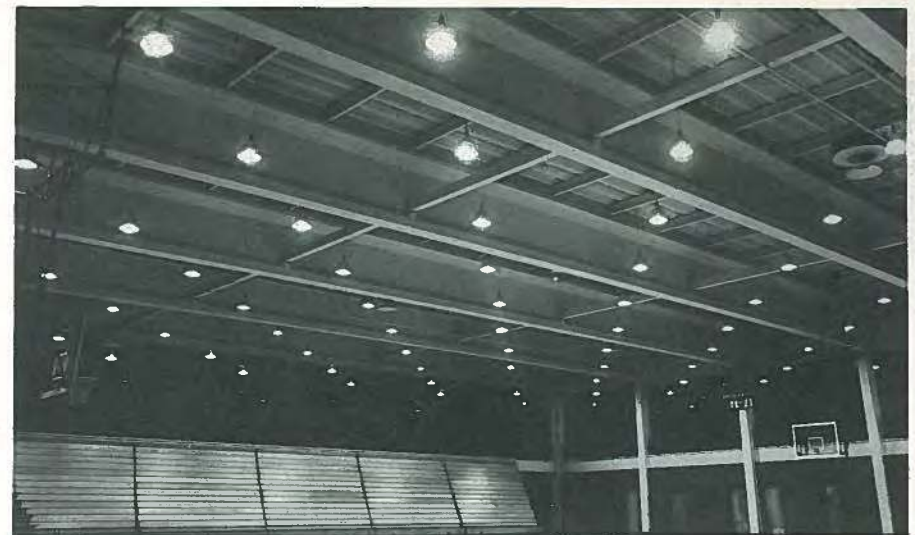
Fig. 42. Completed gymnasium with 120-ft clear span.
