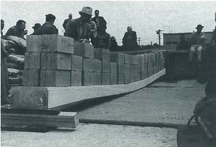
Fig. 6. Load test of prestressed concrete slab.
