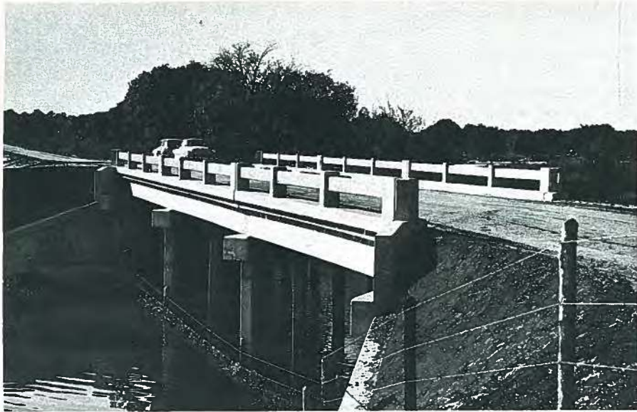
Fig. 15. Precast prestressed county bridge in Sarasota, Florida. Courtesy: Paul Zia.
