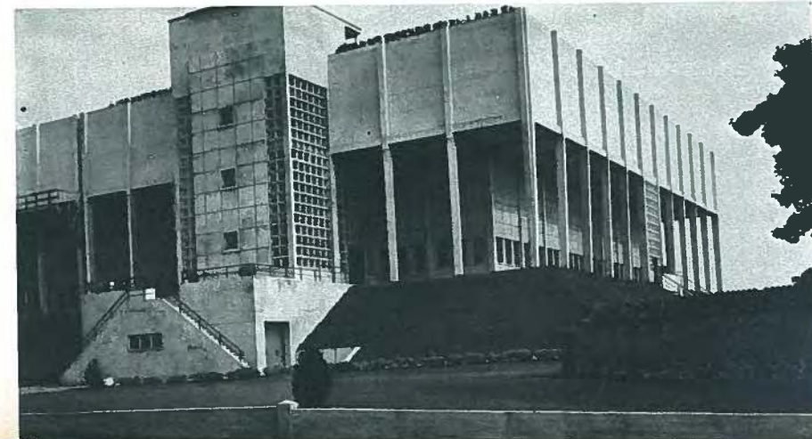
Fig. 31. Water storage reservoir and offices, Orleans, France.
