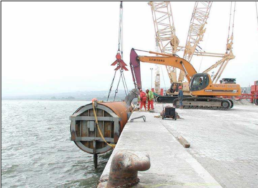
(a) Monopile being floated out to site.
