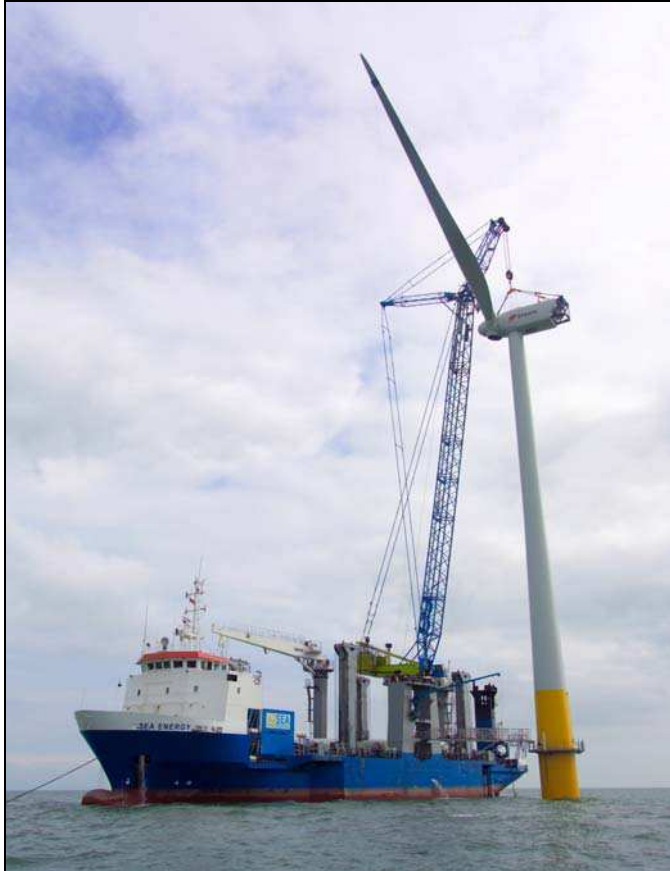
Fig. 22. Wind Turbine being erected with a crane from a special ship at Kentish Flats Offshore Wind Farm, UK (Courtesy: Elsam)
