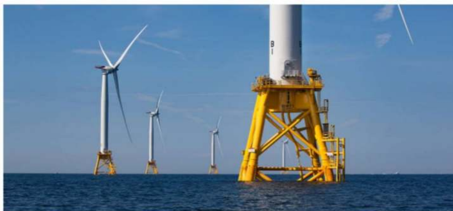
Figure 22. Structures for the Block Island wind farm [159].
