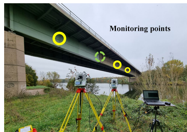
Fig. 10 Exemplary view of two IATS (MoDiTa) on an elongated structure with different forced distances. Here, the observation of a reference point (green dashed line) and simultaneous observation of other monitoring points on the bridge (yellow) are shown
