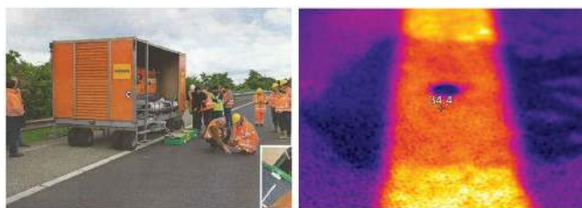
Figure 10. Application of induction heating on Dutch Highway A58.
