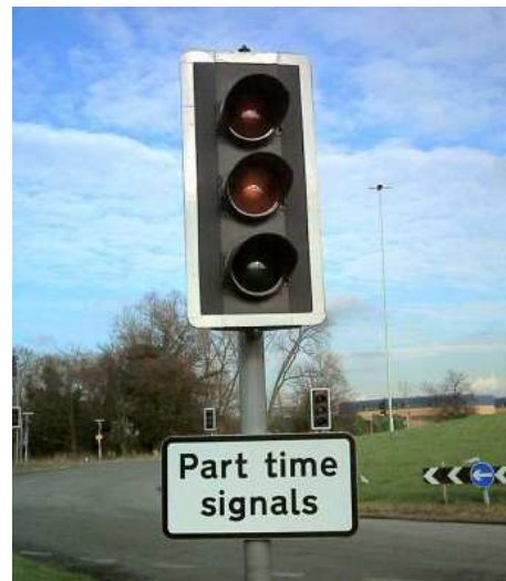
Figure 1: Part time traffic lights are used in many parts of the world to avoid the increased delay that sensor-less signals can introduce during low-traffic hours. The part time warning message is used to avoid people reporting the intentionally turned-off signals as broken (picture reproduced with permission from United Kingdom Roads website: http://www.ukroadsltd.com ).
