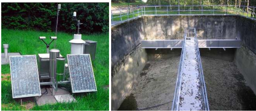
Fig. 1.13 Left: Rain gauge (pluviometer). Right: Stormwater tank.
