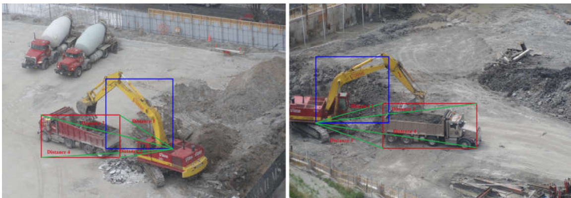
Figure 3: Distances between the corners of trucks and the base point in both left and right configurations
